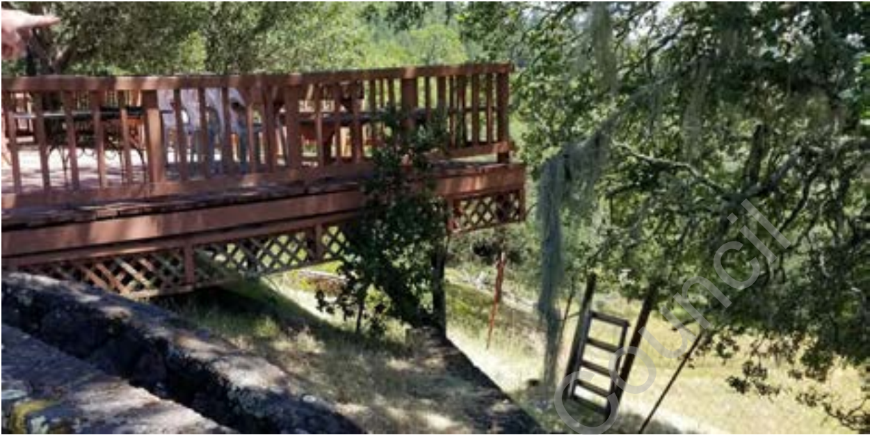
Figure 3. Ignition-prone wood deck
